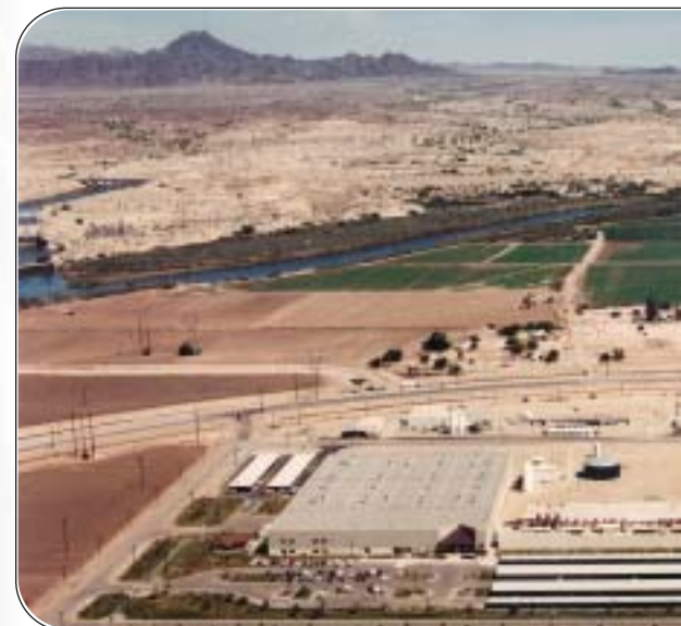
Yuma Desalting Plant; Colorado River in the background.
