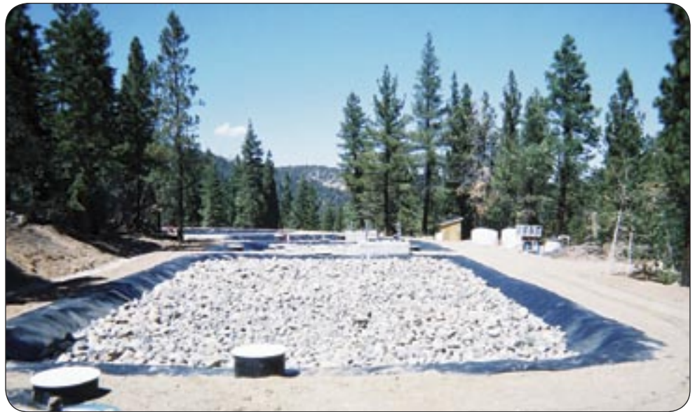
The compost-free bioreactor at the Leviathan Mine treats up to 30 gallon per minute ARD flow year round before releasing it to Aspen Creek.
