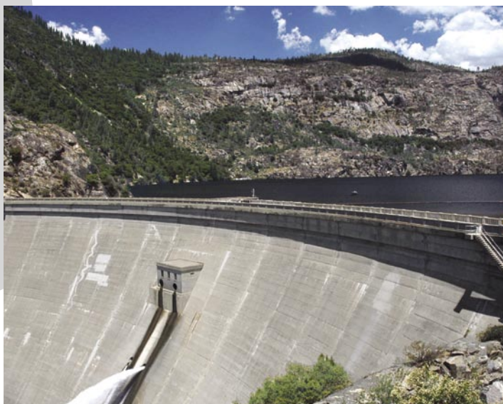
O'Shaughnessy Dam in Hetch Hetchy Valley.
