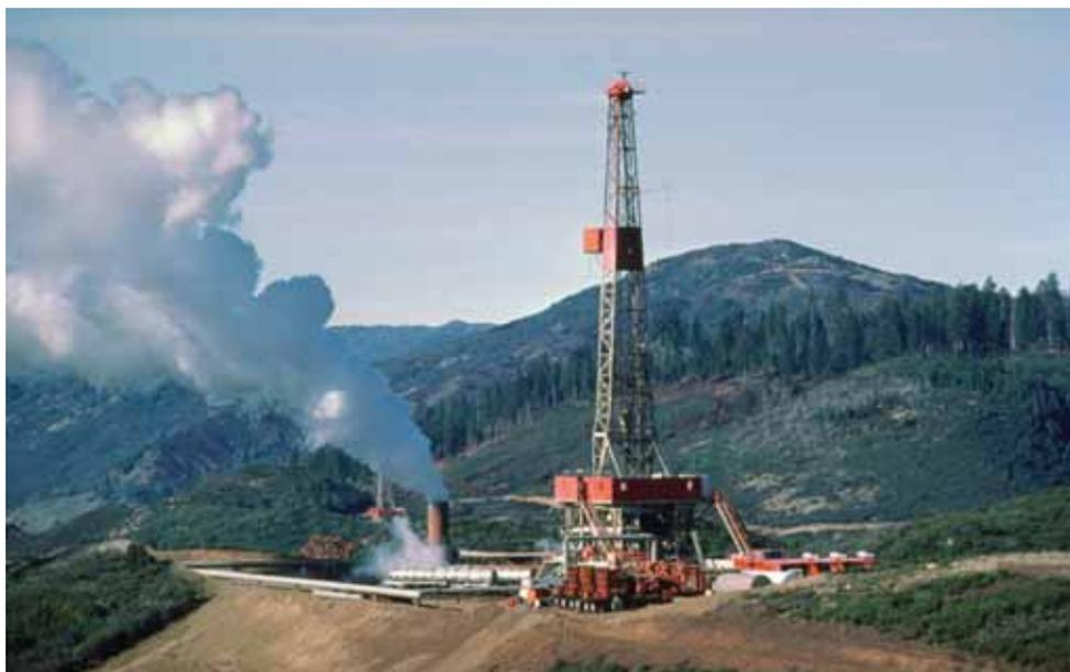
Drilling a well for injection of Santa Rosa's recycled wastewater to improve steam generation at The Geysers.
