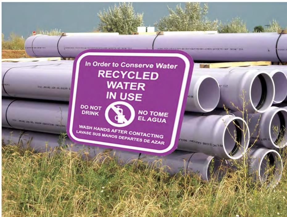
development of a dual, parallel pipe system consisting of a potable waterline and a purple nonpotable irrigation waterline. Currently, ACWWA has over 28 miles of nonpotable distribution piping in place that provides irrigation for nearly 30 percent of the service area. Ultimately, over 59 miles of purple nonpotable piping is proposed. This water conservation effort comprises a significant proportion of the agency's overall water portfolio.
